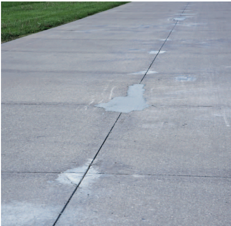
The taxiway after repair.
