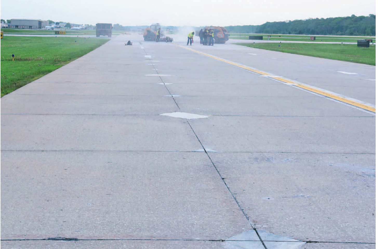
Completed repairs on taxiway using TechCrete.
