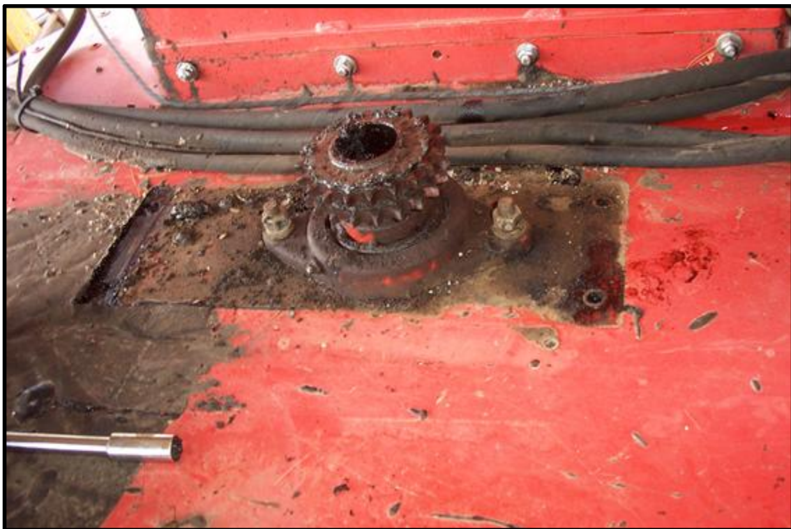
Fig. 6-4 Removal of Motor Mount Assembly
