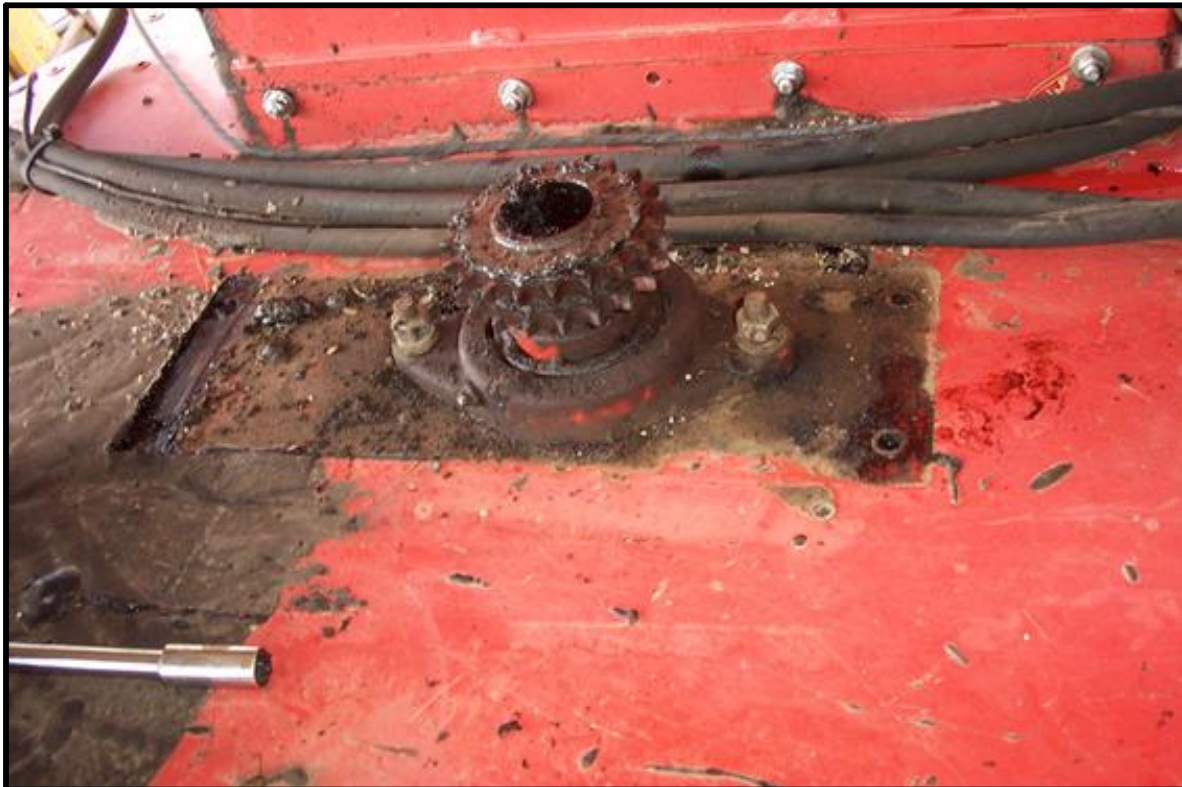
Fig. 6-5 Removal of Motor Mount Assembly
