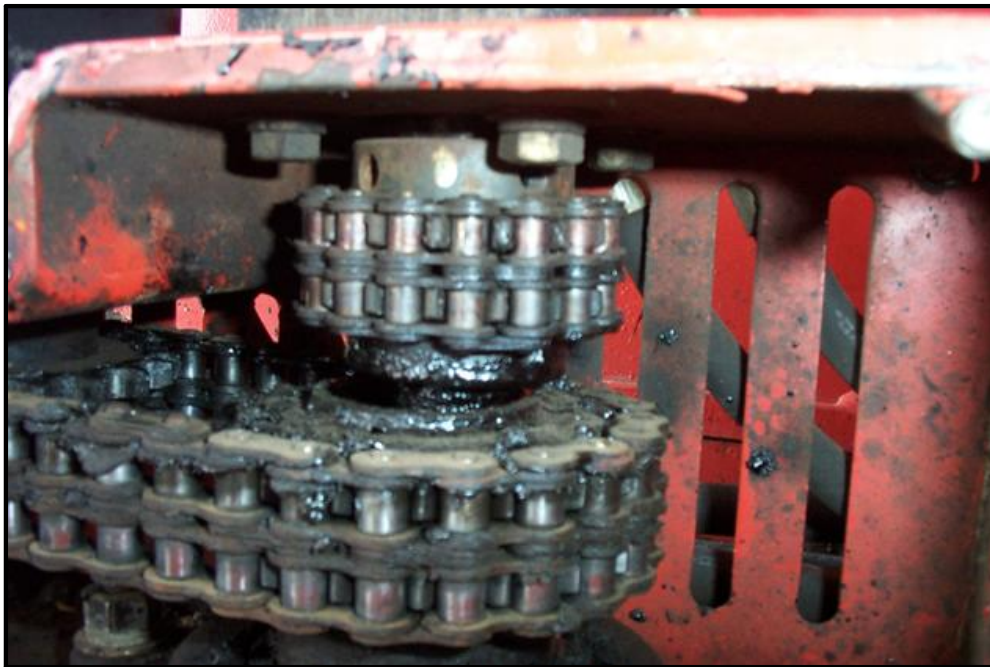
Fig. 6-4 Agitator and Pump Shaft Alignment
